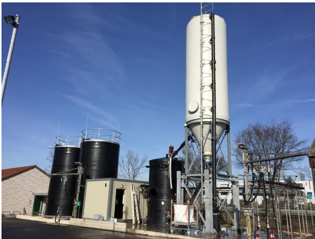
Figure 9: Brine production system with salt silo and brine storage tanks at the highways maintenance center Erlangen on the A3 (Die Autobahn GmbH, Germany)
